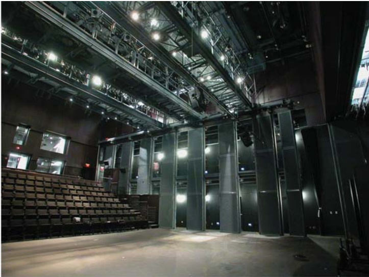
VIEW FROM STAGE (VARIABLE ACOUSTICS OPENED, ABSORPTIVE SURFACE EXPOSED)
